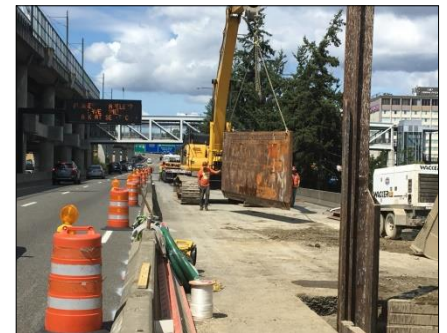
Lane Closure - Utility Excavation
