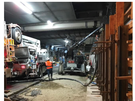
West Wall Seismic Reinforcement
